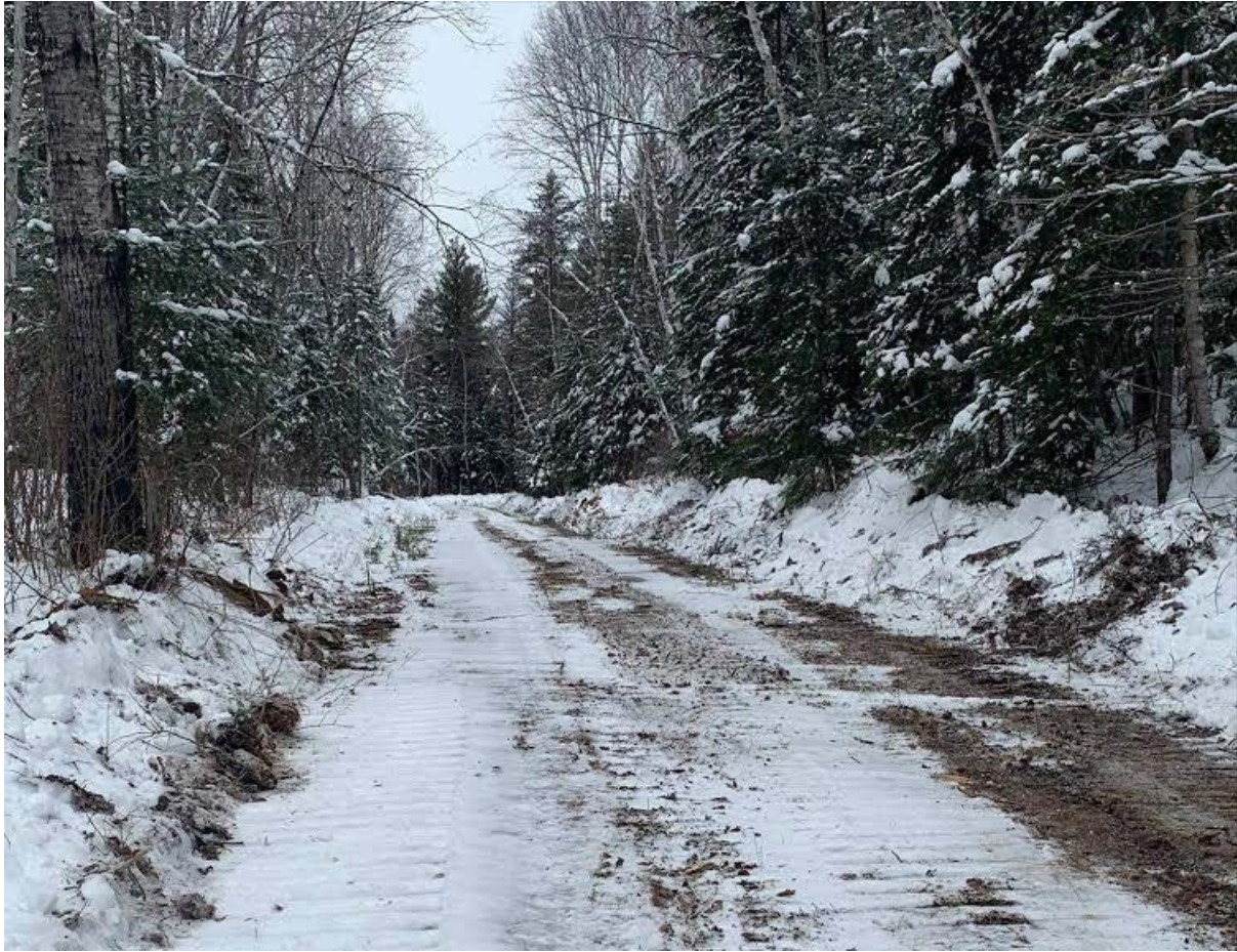
Figure 4: Road clearing underway at Edleston
